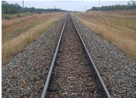
Initial Railway Track
