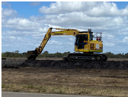
Excavator Distributing Material
