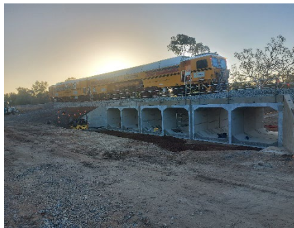
Completed Culverts and Bridge
