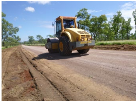
Rolling for compaction
