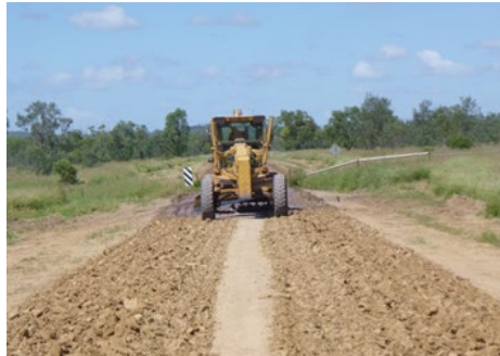
Tying for Heavy Formation Grade
